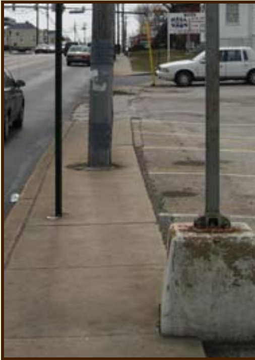
Utility Poles and Signs Limit Pedestrian Mobility
