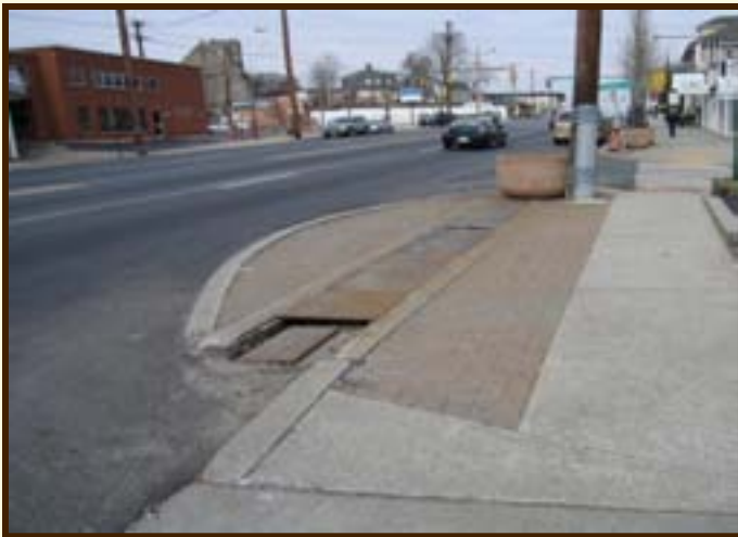
Current Drainage Channel
